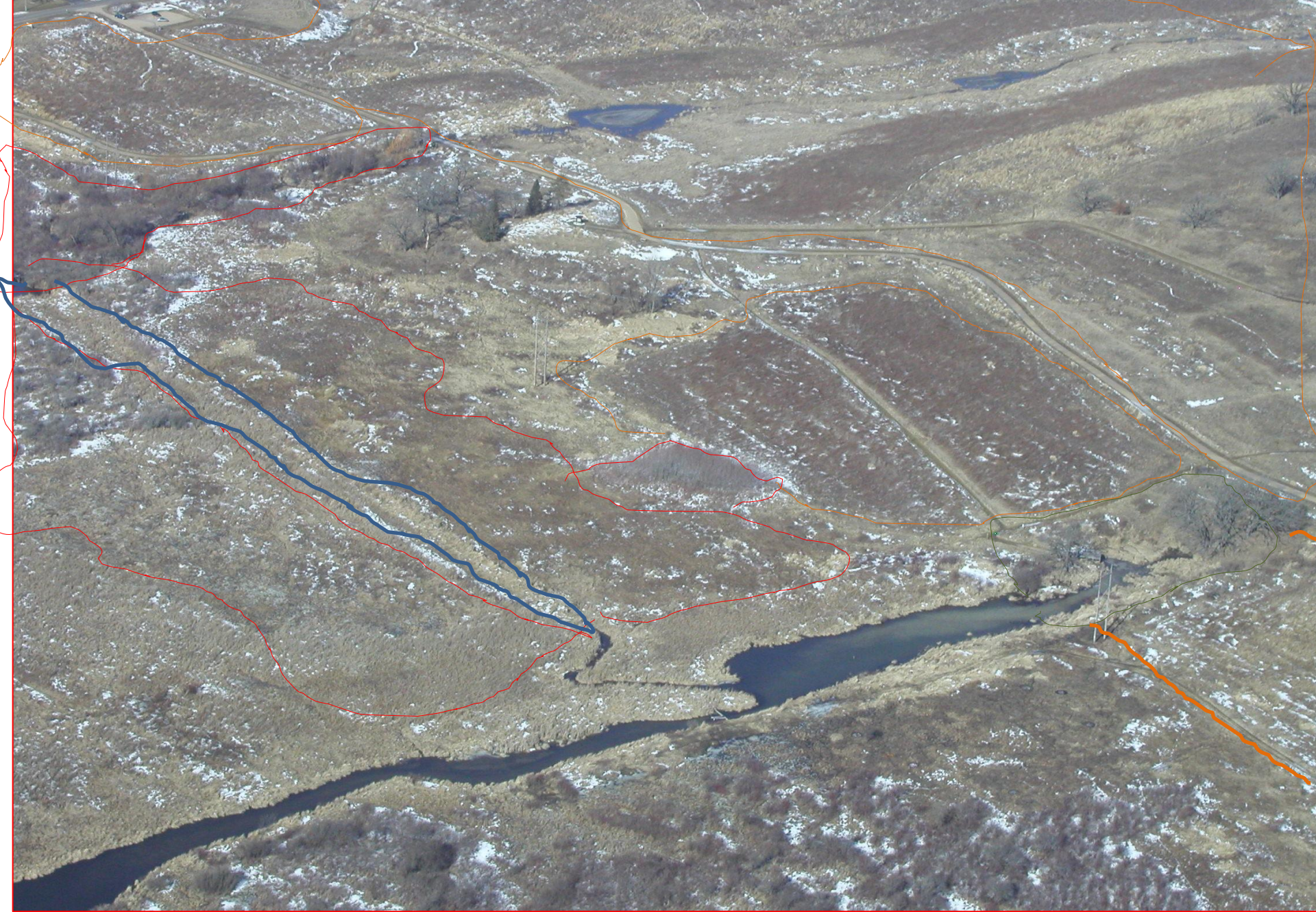
Ditch Fill and Sediment Basins Winter 2004
