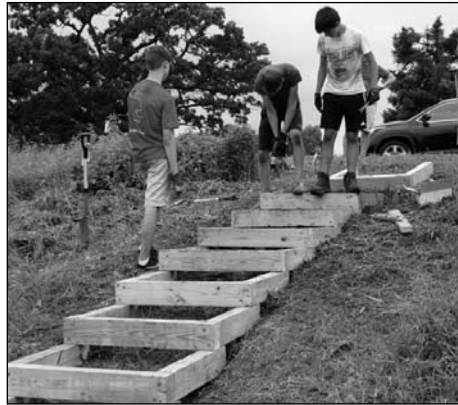
Construction of the homestead site steps
