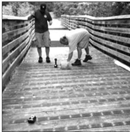
Mark Warshauer and city employee Dennis Hellenbrand install friction strips
