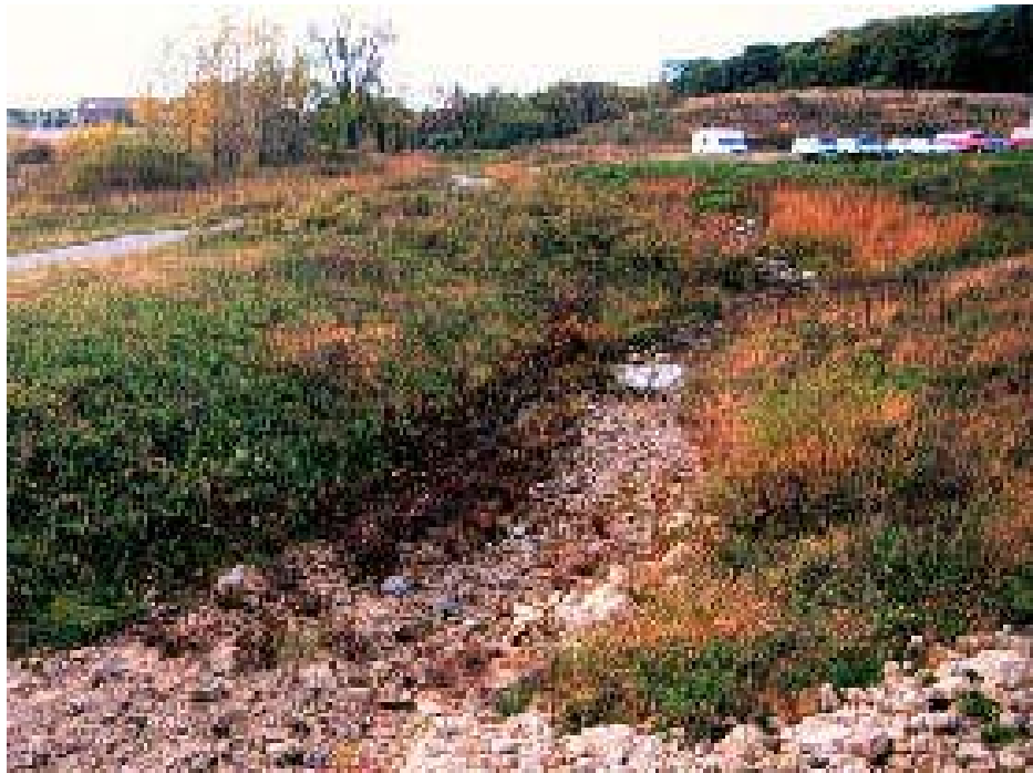
The dry bed of the South Fork Channel between Old Sauk Road and University Avenue
