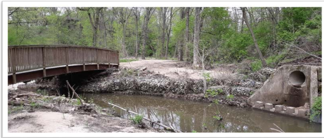
Figure 42: Upstream face of Bridge #5
