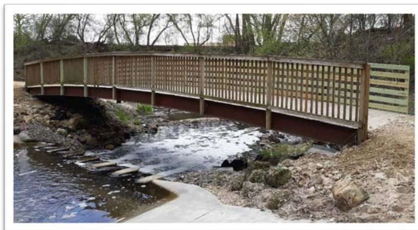
Figure 38: Upstream face of Bridge #1
