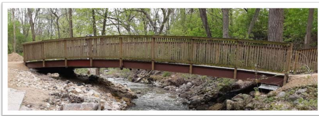
Figure 43: Upstream face of Bridge #6
