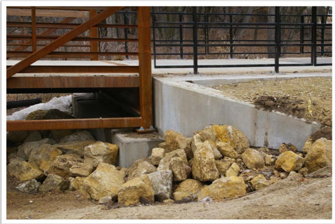
Figure 49: Example bridge concrete footing abutment substructure
