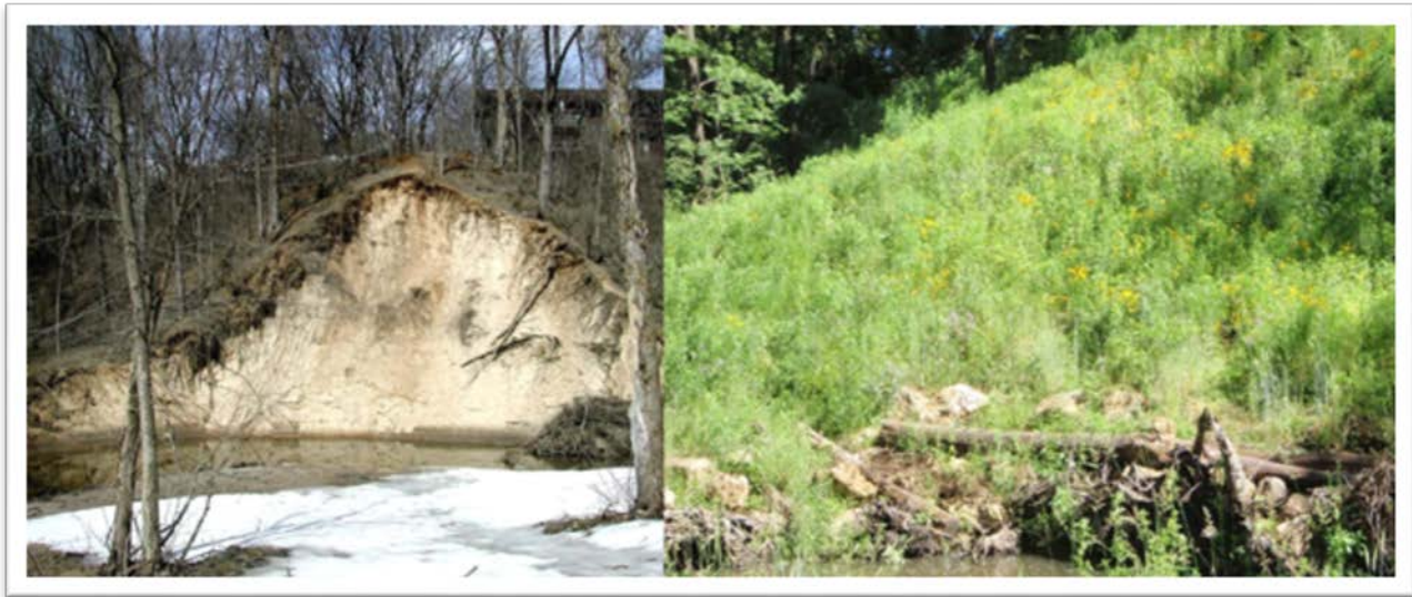
Figure 2: Photo of eroded slope adjacent to Pheasant Branch between Park Street and Century Avenue in 2005 (left) and same slope after construction taken in 2009 (right).
