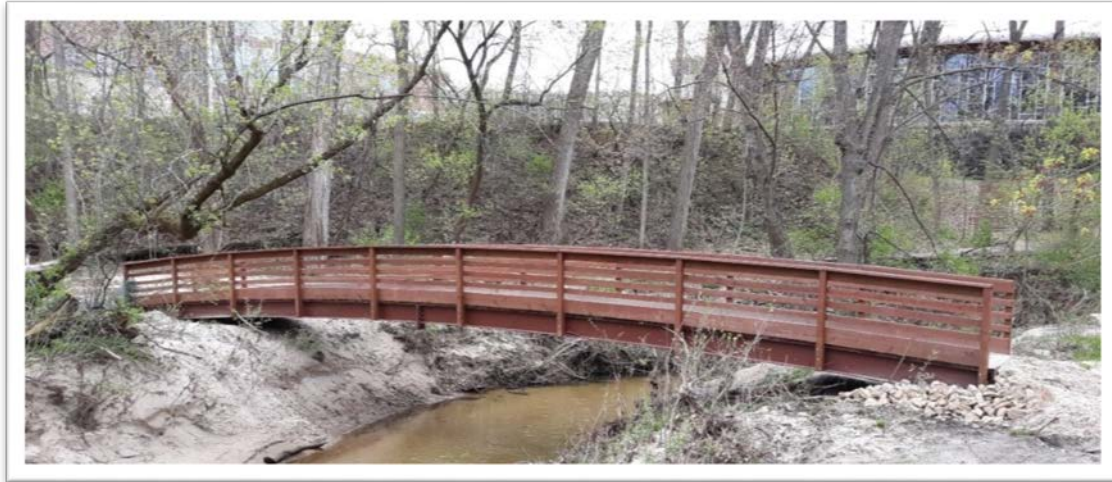
Figure 40: Upstream face of Bridge #3
