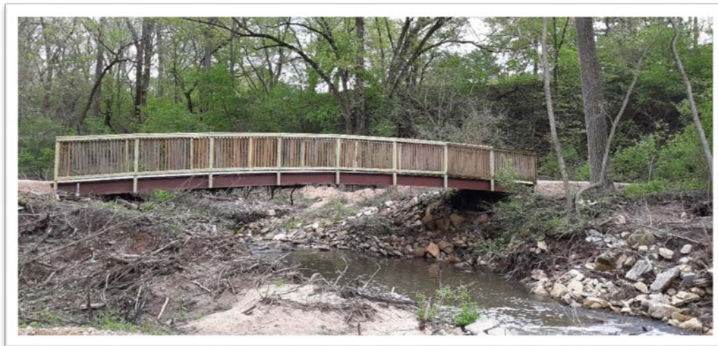
Figure 41: Upstream face of Bridge #4
