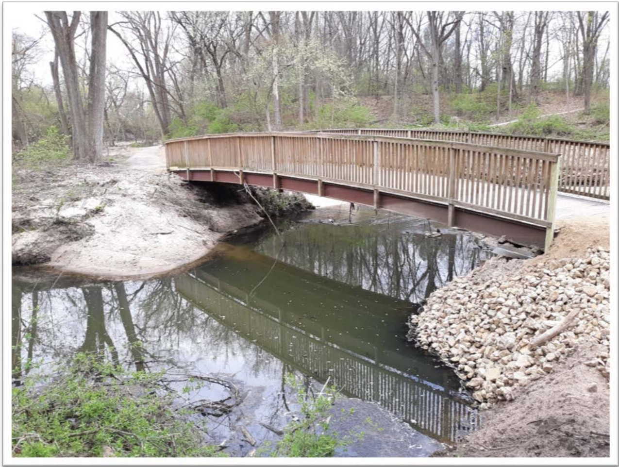
Figure 39: Upstream face of Bridge #2
