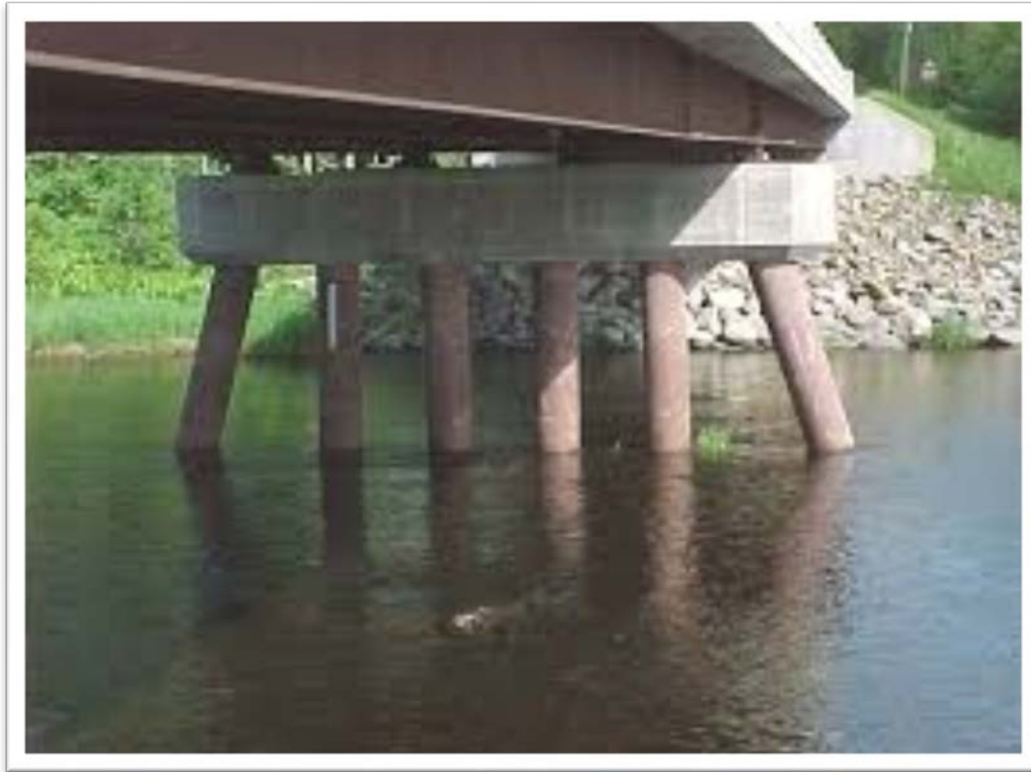
Figure 50: Example bridge bent pile pier substructure
