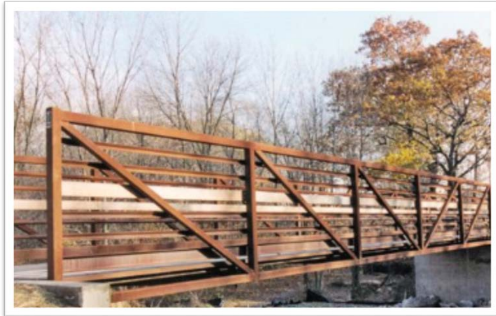
Figure 47: Example bridge railing style
