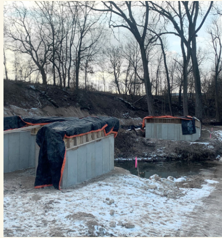
Stabilization and restoration work in the creek corridor
